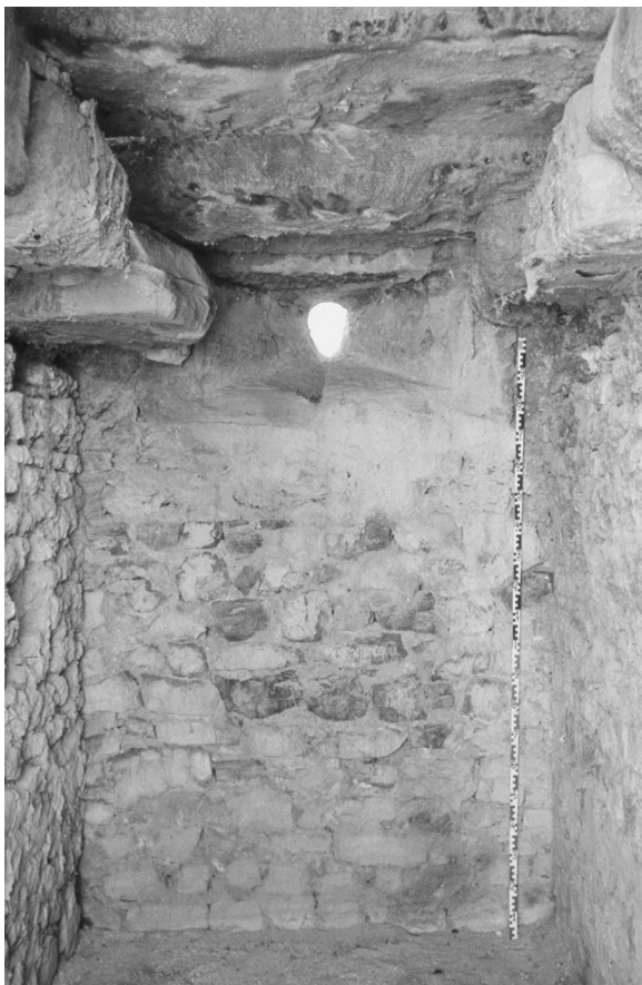
FIGURE 9. Cell B, looking south toward one of the three extant embrasures. Photograph Friedrich Rakob. (Negative D-DAI-ROM-NA-RAK-37538)
